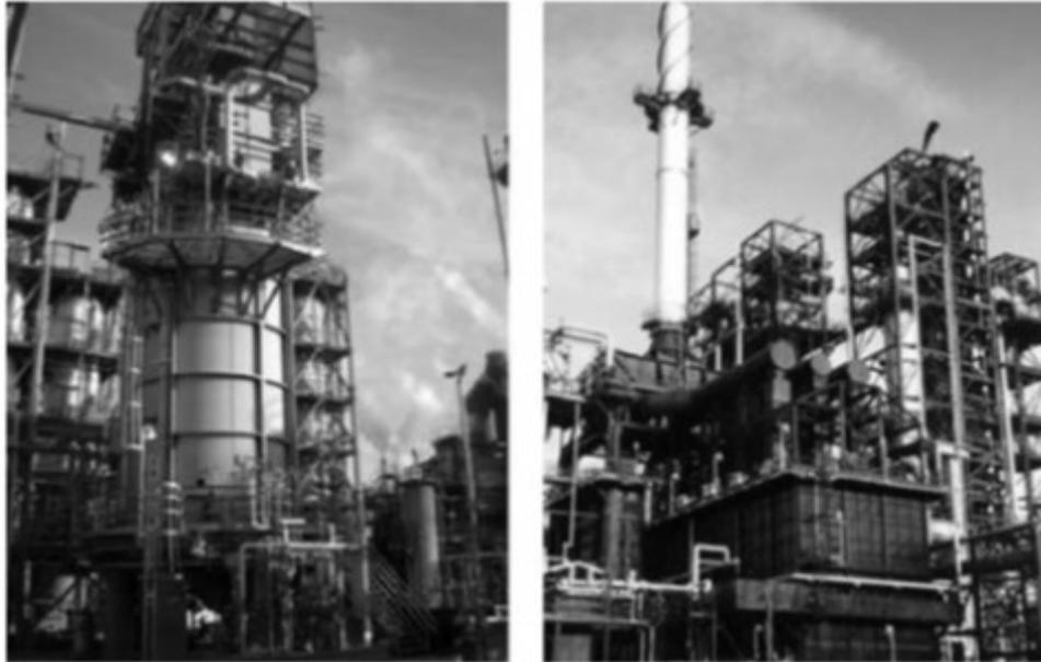
**Figure 1:** Two types of refinery heater showing a cylindrical heater (left) and a cabin heater (photos provided courtesy of Born Heaters, Canada, an Onquest Company)
